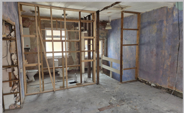
First Floor Frame Work
