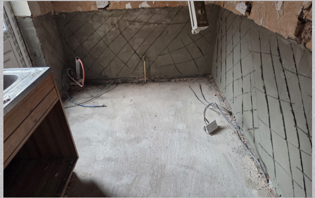
Kitchen (Damp Works)
